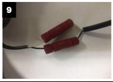
Attach the wires of the trim ring harness with the (2) Posi-Lock™ connectors to the trim ring wires. White wire to white wire. Black wire to black wire.
