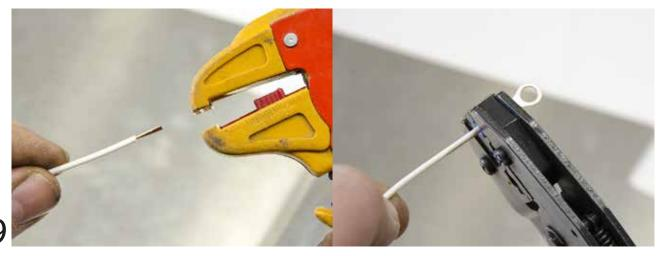
Strip cable provided and attach ring connector. Attention: If you can combine the ground cables of the indicators.
